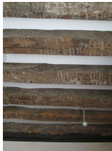
Floor joists of the first floor Hall
