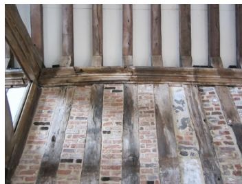
Studs with brick infill
