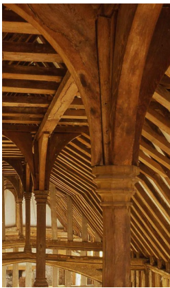
The crown post roof
