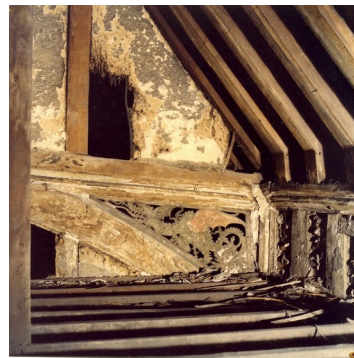
The dragon in the attic
