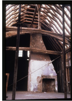
A chimney in the middle of the Hall
